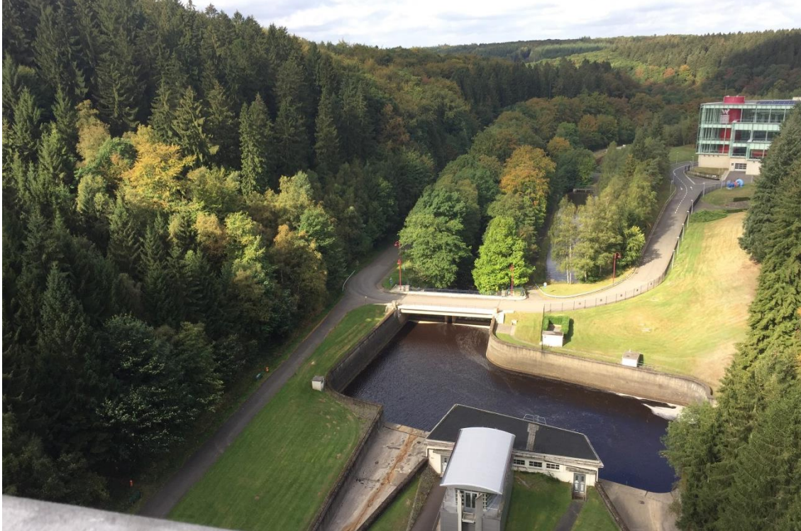
Photo 1: Water treatment plant in Verviers (SWDE)
